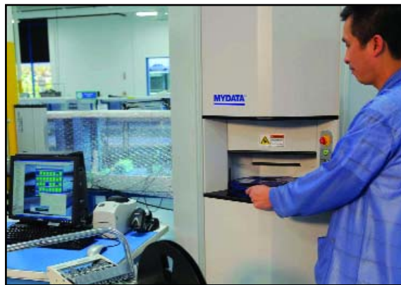
SMT lines also include component towers which select components based on system requests and provide humidity-controlled storage for moisture-sensitive parts.
